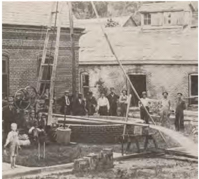
The water supply was obtained from a well just east of the building, 20' deep and 12' in diameter. The water was "unexcelled anywhere for domestic purposes being clear, sparkling, and chemically pure."
